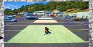
Cool pavements on parking spot near Yogeshwar Society and Mansata Industrial Area
